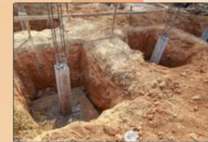
Ground preparation for foundation works and confirmation of foundation conditions
