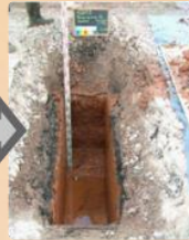
Geotechnical test pit excavation to inform design and depth of foundations
