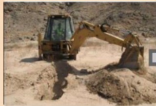
Geotechnical test pit excavation to inform design and depth of foundations
