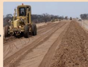
Placement and compaction of tested and verified road building material
