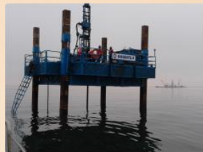
Offshore geotechnical drilling in Walvis Bay Harbour
